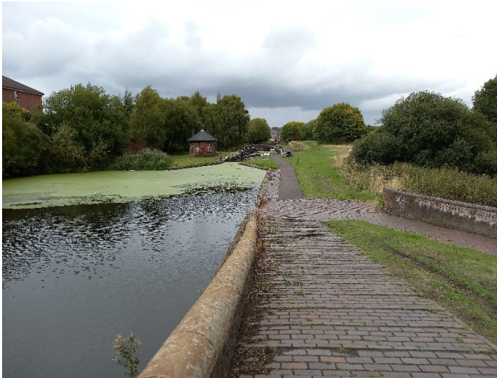
Figure 2.12 Canal side cycle provision
