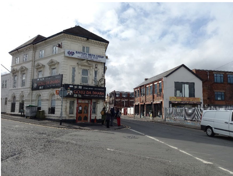
Figure 2.11 New Street / Rolfe Street junction (gateway to Rolfe Street)
