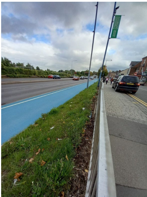
Figure 2.13 A457 Cycle Lane (phase 2 extension under construction)
